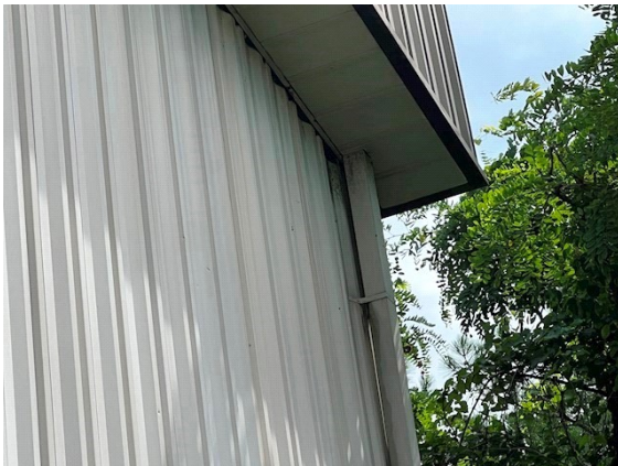
Parapet Wall System: Downspout connected to gutter inside parapet wall
