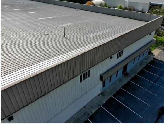
Parapet Wall System: Aerial view of parapet wall.
