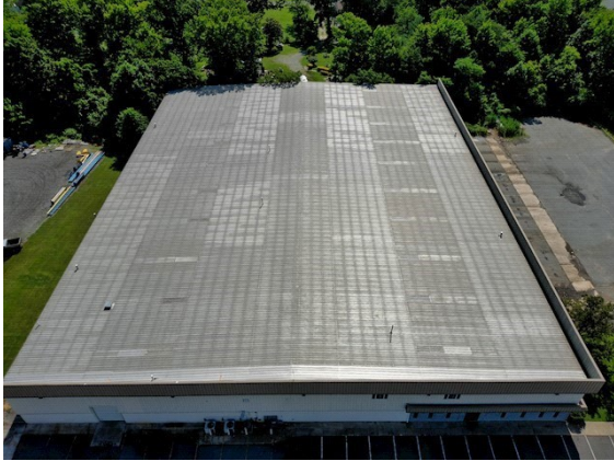
Roofing: Birdseye view of entire roof covering looking east
