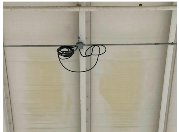
Roof Insulation: Electrical cable for since removed equipment
