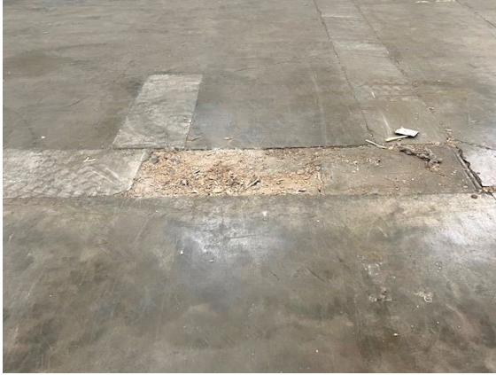
Floor / Slab: Patch and seal
