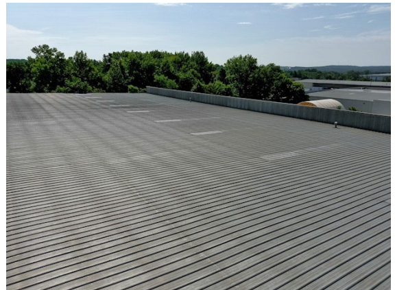
Roofing: View of southern parapet wall
