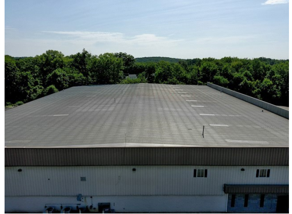
Roofing: Oblique view of roof covering looking east
