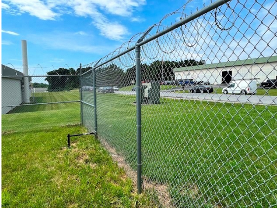
Fences / Enclosures: Fencing in good condition
