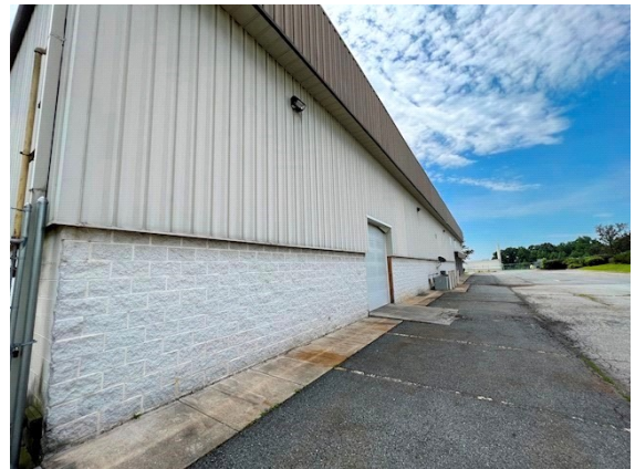
Grading / Drainage: Positive slope away from west side of building
