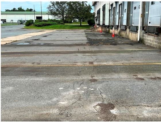
Grading / Drainage: Near level grading in dock/loading area
