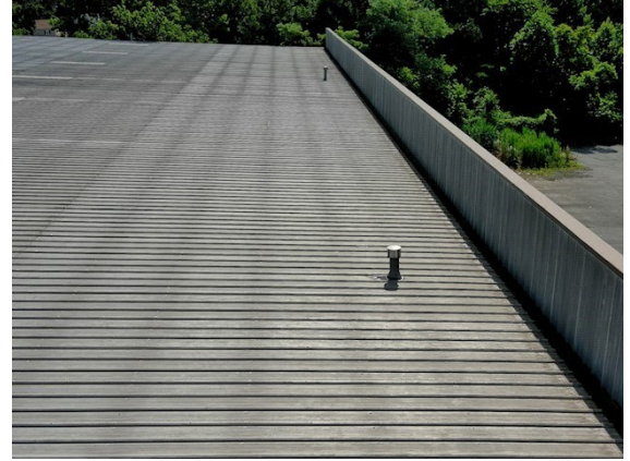
Parapet Wall System: Parapet wall along southern side of roof
