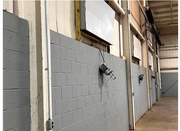
Interior Foundation: Concrete block foundation/wall in good condition
